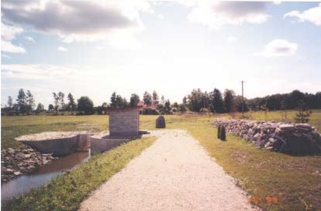
Figure 5. The Rägina water monitoring station.
