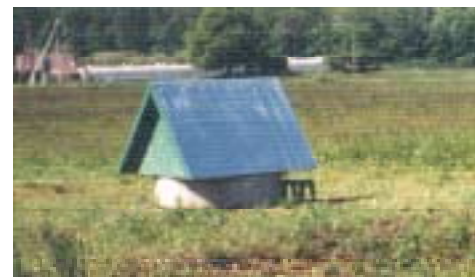
Fig. 2. Well with tin-covered roof
