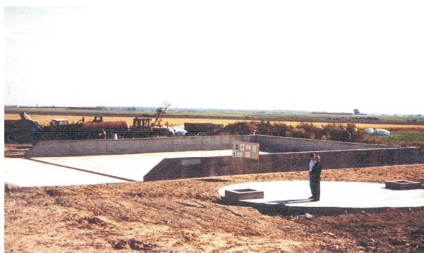
Figure 1. Manure storage and urine reservoir on V. Liutkevicius farm in Kedainiai district.
